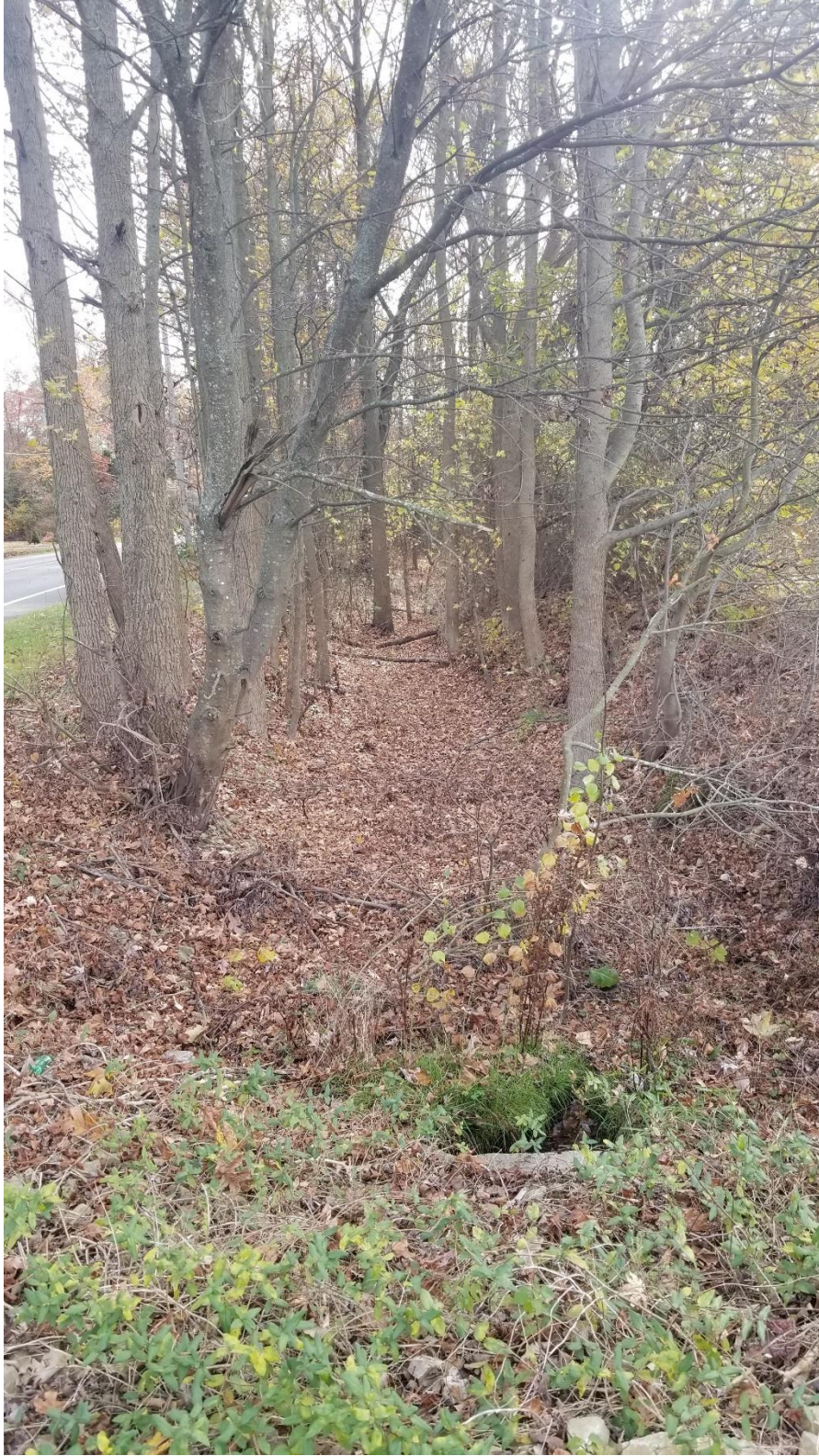
Photo 16 – Standing along Buck Road, across the street of the site, standing uphill of the existing pipe outfall looking south.
